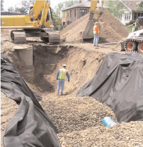
Nebraska Avenue trenches under construction, 2006
