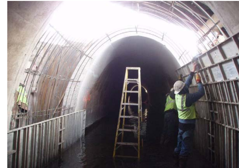
Creation of concrete forms to connect old sewer sections to new
