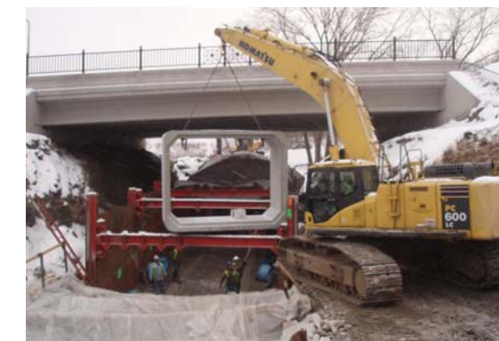
Installation of new sections of storm sewer under L'Orient Avenue Bridge
