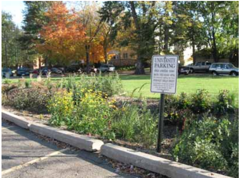
The garden receives runoff from a 6000' parking lot
