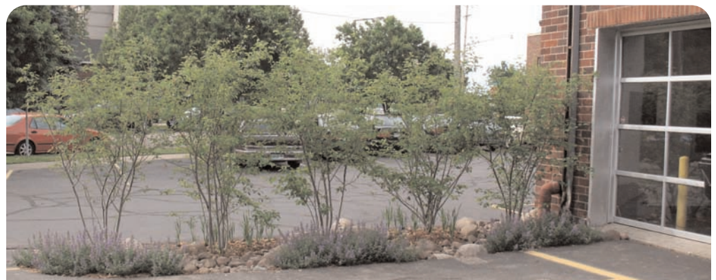
This parking lot raingarden receives roof and surface runoff.
