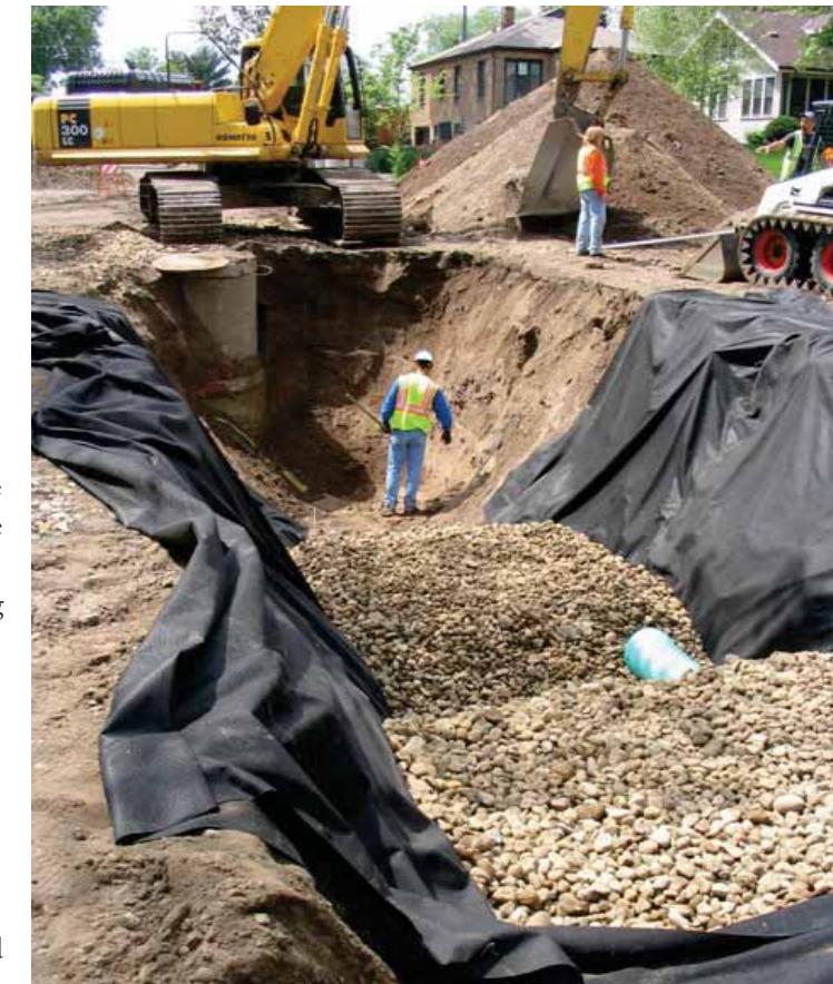
In-street trench under construction
