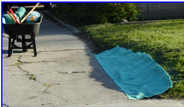
Example of wood fiber mulch blanket
