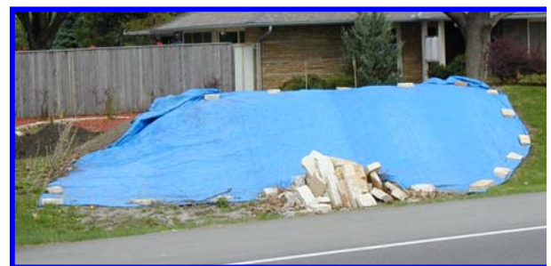
Tarp Covering Soil Stockpile
