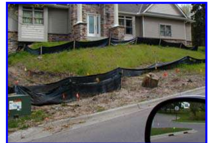
Silt Fence with Seeding
