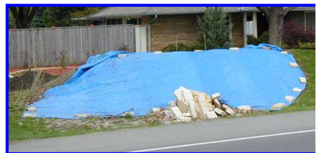
Tarp Covering Soil Stockpile
