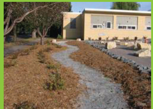
Shown during construction (top) and after completion, this rain garden captures roof and parking lot runoff.
