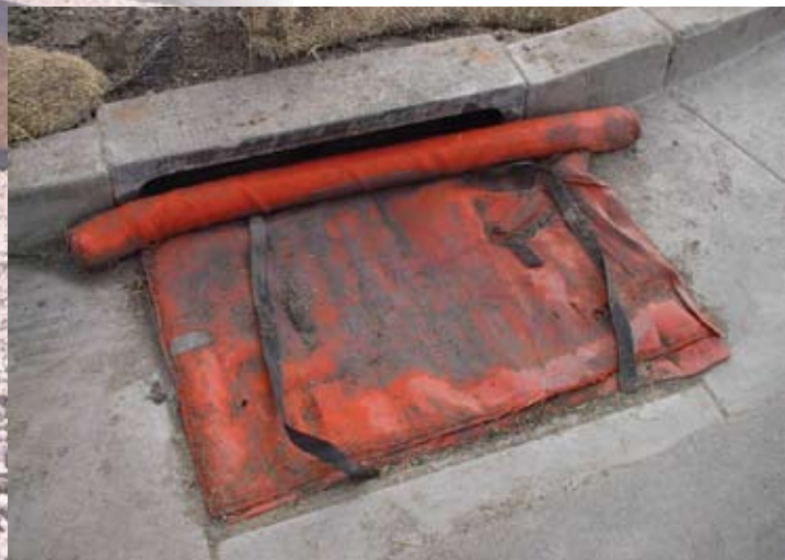
A storm drain inlet protected from runoff at a construction site.
