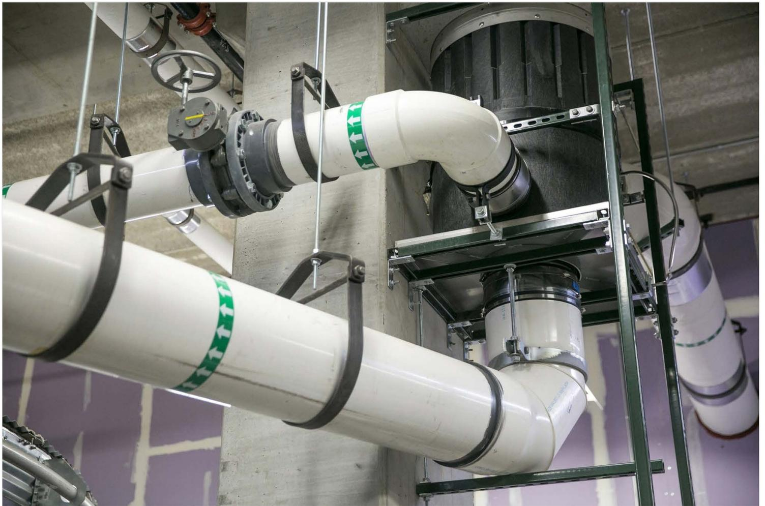
Inside CHS Field, one pipe brings in water from the roof, another puts filtered water into a 27,000 gallon cistern, and a third puts filtered debris back into the storm drain system. *Evan Frost | MPR News*
