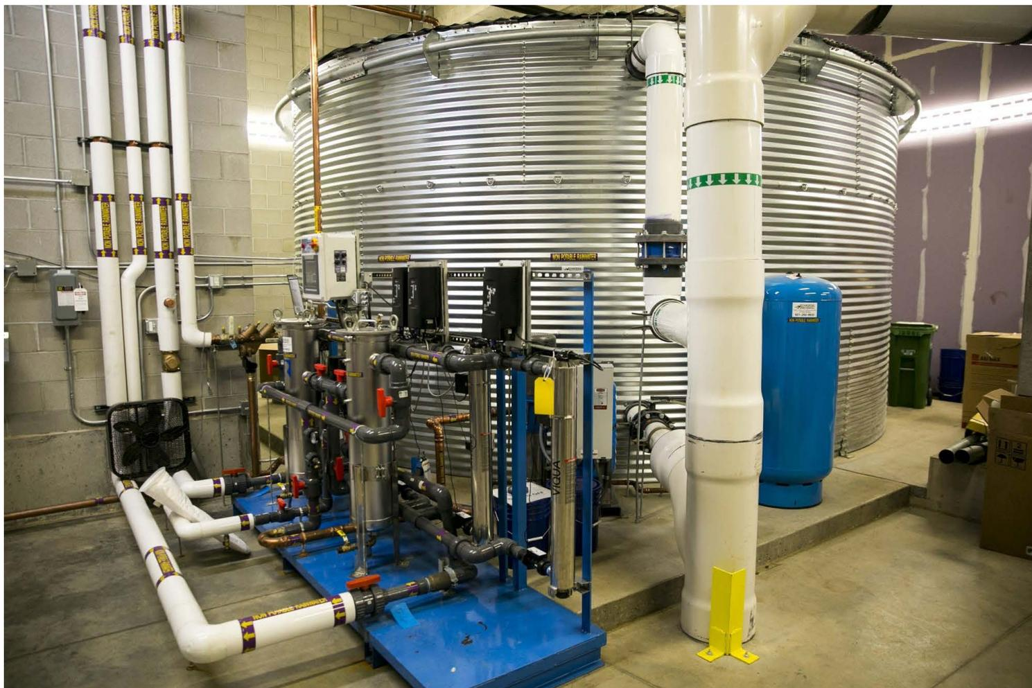
A 27,000 gallon cistern designed to hold rainwater sits empty for the winter inside CHS Field. The rainwater harvesting system collects water that falls on the roof of the facilities, then treats it and uses it for irrigation and toilet flushing. *Evan Frost | MPR News*
