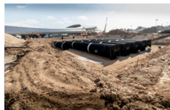
Rainwater harvesting and reuse at Allianz Field (Image credit: Sara Rubinstein)
