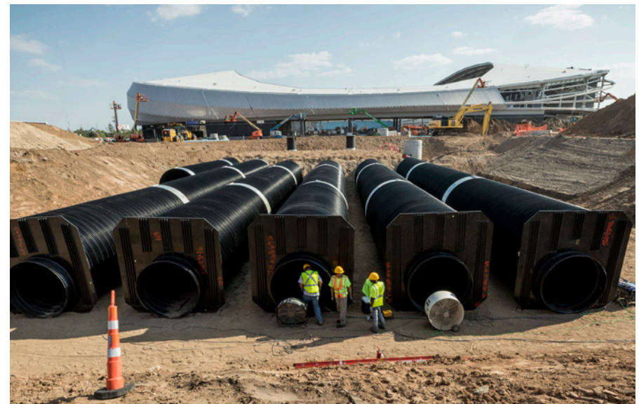
Water collection and reuse system at Allianz Field
