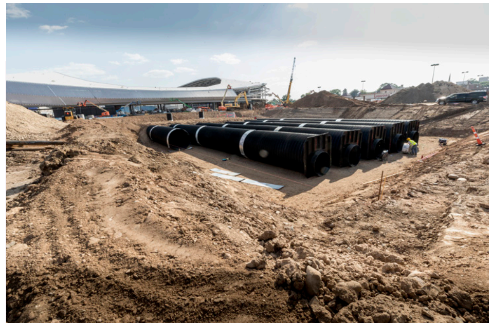
Rainwater collection and reuse system at Allianz Field
