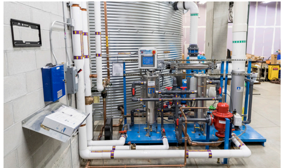
CHS Field cistern collects rainwater to irrigate the field.
