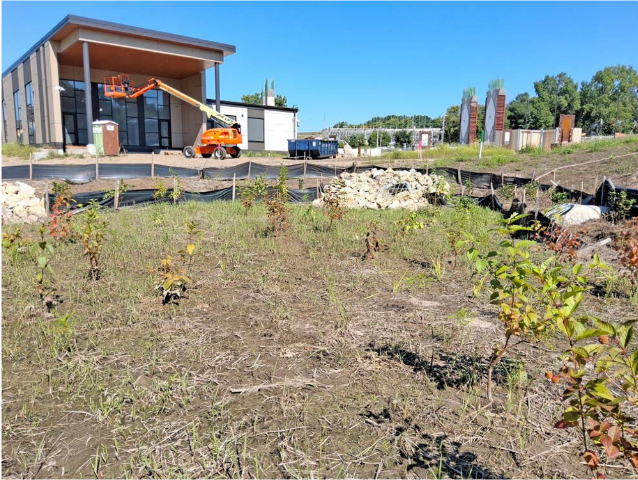
Construction of the Waqan Típi Center.
