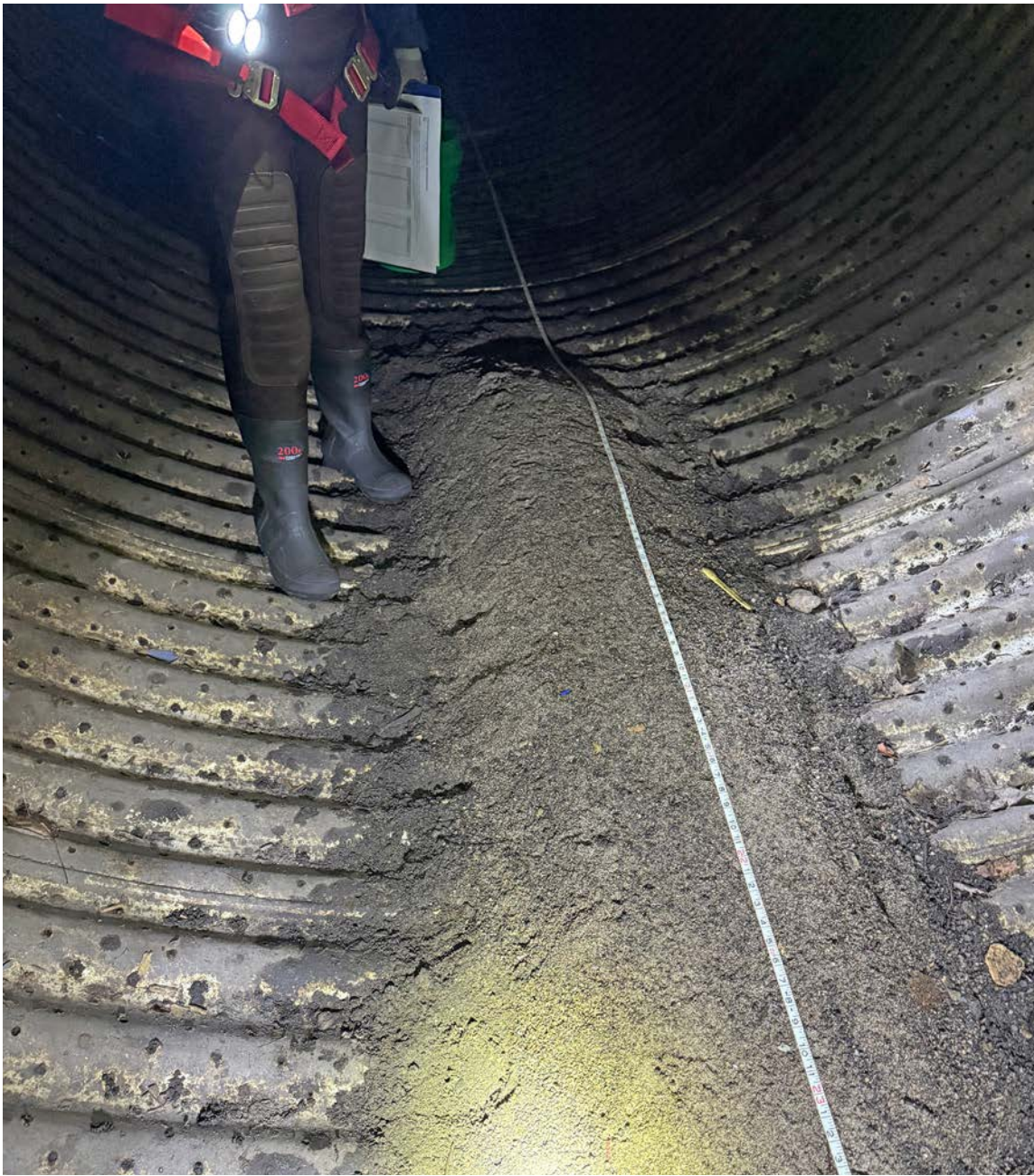
Inspecting the pipe gallery at AHUG, an underground infiltration system.
