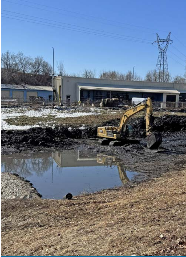
Pooled BMP pond dredging at Atwater Western Pond.
