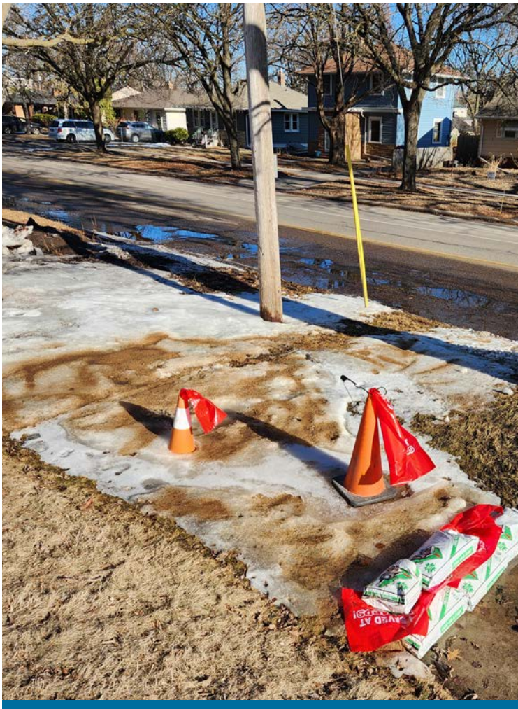
Groundwater flow on sidewalks and roadways causes icy conditions.
