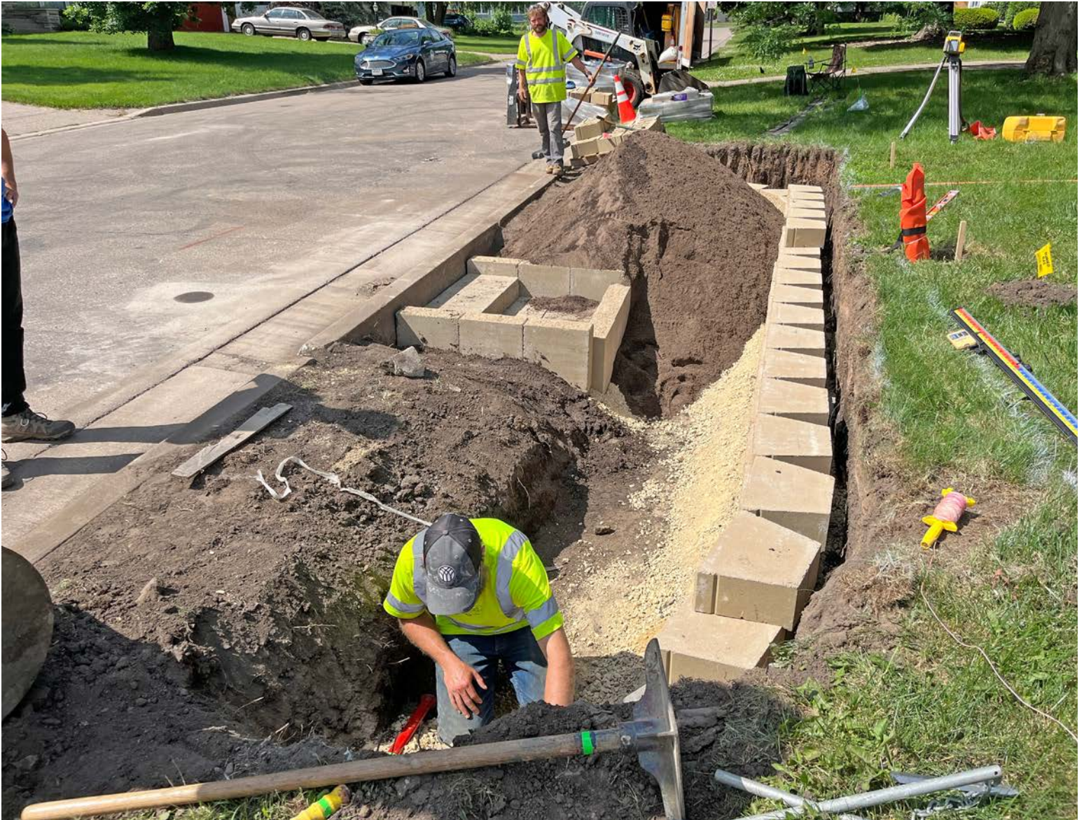
Boulevard rain garden during construction.
