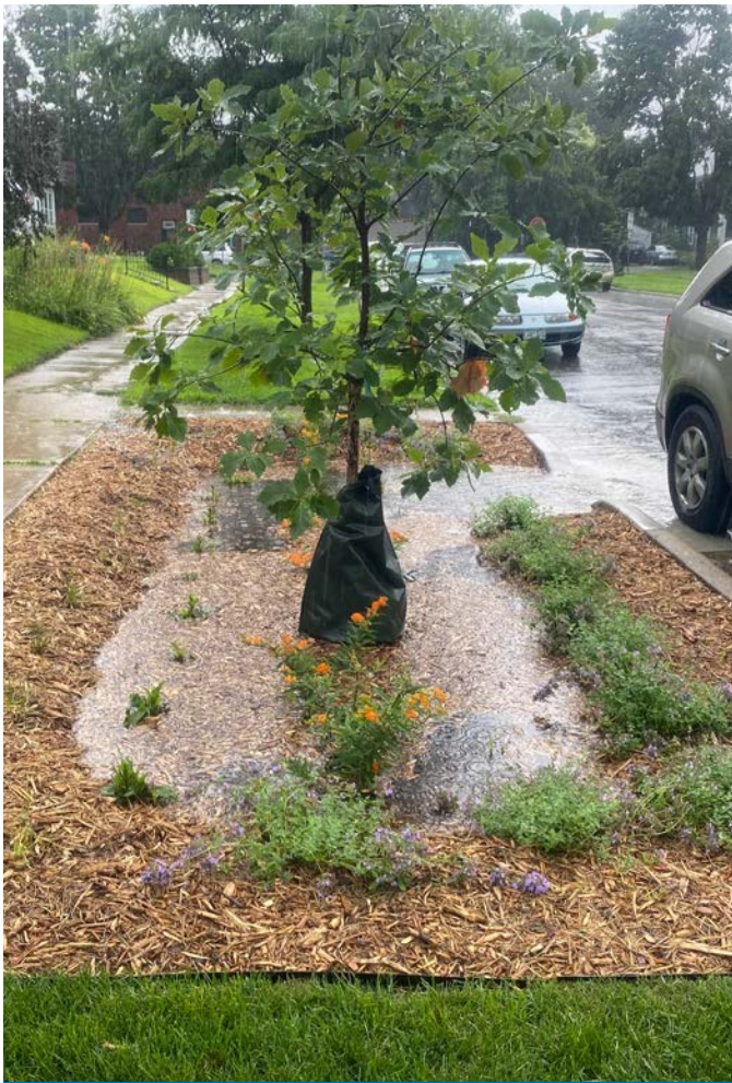
Boulevard rain garden collecting stormwater runoff as designed.
