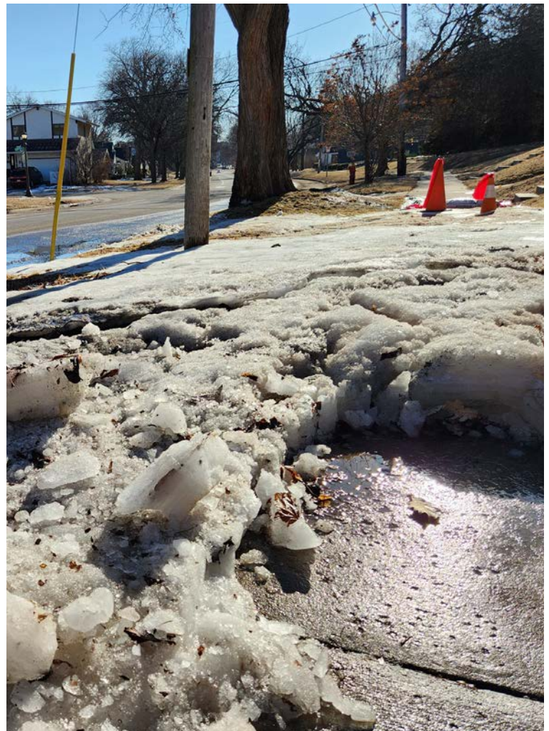
Ice buildup on sidewalk from groundwater flow.
