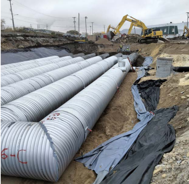
Installing required permanent underground stormwater treatment.
